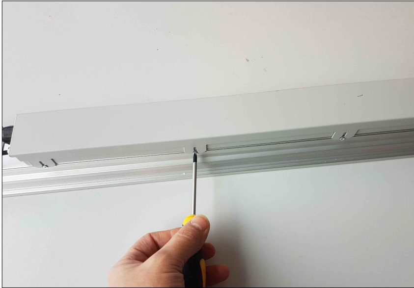
3) loosen screw connection of driver housing
